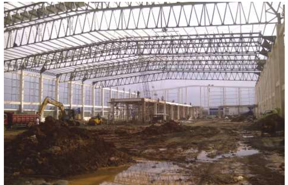
PROYEK : FACTORY 2 – PT.GS BATTERY SEMARANG
