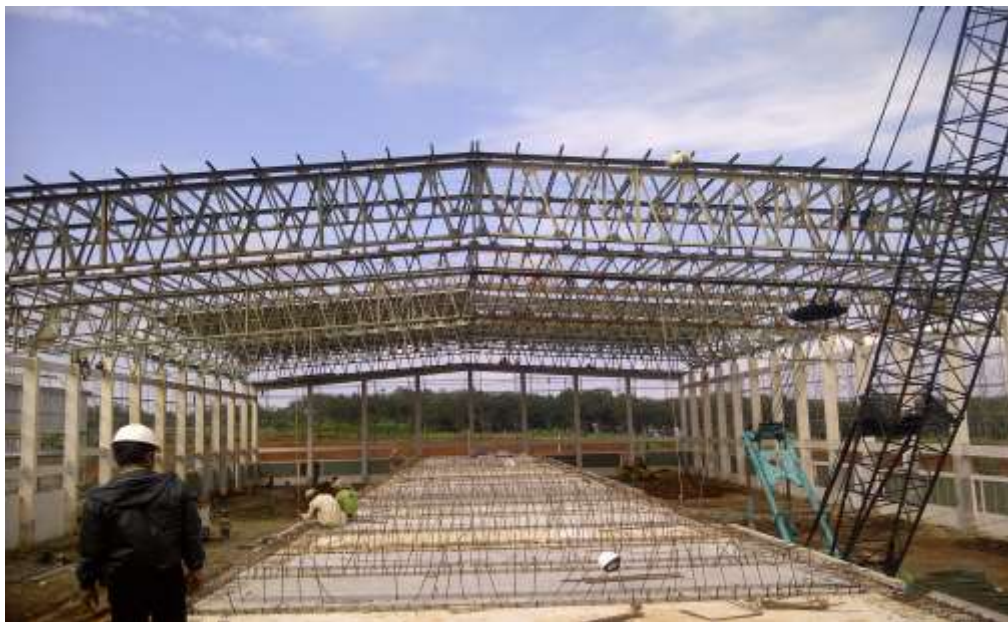
PROYEK : FACTORY 2 – PT.GS BATTERY SEMARANG
